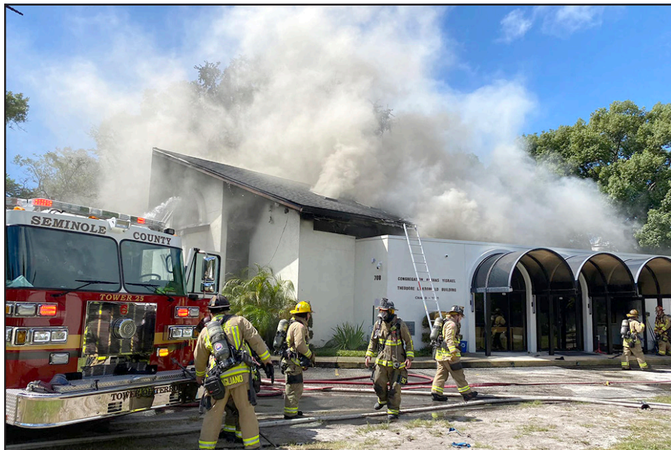
Firefighters work to put out the fire at Chabad of Greater Orlando.
